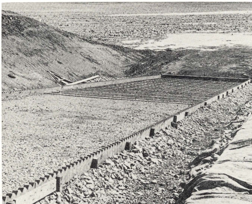
Boat ramp under construction at John Redmond Reservoir.
